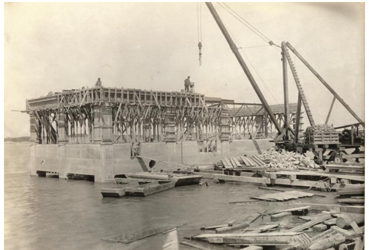
Building the Pump House MCS Photo P2442
