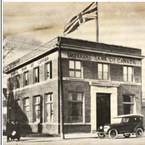
The new bank building, 1921 MCS P308
